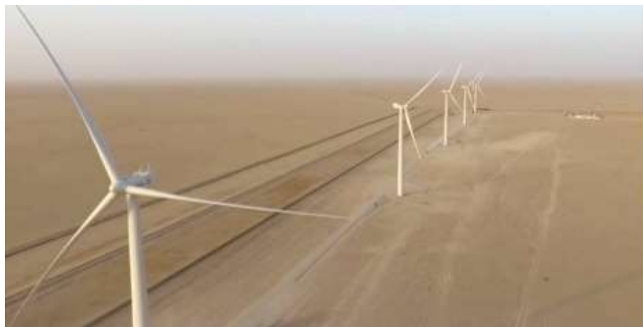
Figure (5-3) :Shagaya (phase I) 10 MW wind turbines, total of 5 wind turbines each of 2 MW.
