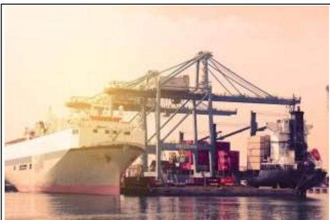
Figure 1-33: Shuwaikh seaport. (Source: Kuwait Ports Authority website)
